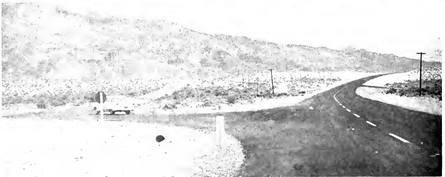
UPPER Looking northwesterly from end of project. Old highway to the right with new crossing of the Southern Pacific Railroad narrow-gauge tracks to the left. CENTER Beginning of job looking easterly from junction with US 6/395. LOWER Looking easterly showing junction of old and new alignments.
